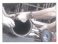
Step 5: Slowly rotate the CheckMate<sup>TM</sup> Valve, as you continue to press the rubber tape into place around the circumference of the valve. As you apply more of the tape, press it firmly into place and line the edge of the tape up with the edge of the valve.
