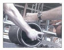
**Step 3:** Unroll a small amount of the 1/8" thick vulcanized rubber tape. Remove plastic from both sides of the unrolled tape. Leave length of tape attached to roll.
