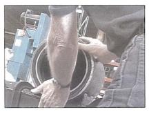
Step 10: If you have removed the CheckMate<sup>TM</sup> Valve to apply another layer of rubber tape, gently place the CheckMate<sup>TM</sup> Valve back into the pipe. There should be no rolling or moving of the rubber tape as you slide the valve into place. The valve should fit snugly into the pipe with the area of the valve marked top at the 12:00 position.
