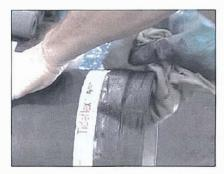
Step 1: Clean the outside surface on the clamped end of the CheckMate<sup>TM</sup> Valve. Remove all surface dirt so the 1/8" vulcanized rubber tape will stick to the valve.
