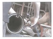
Step 7: When the O.D. reaches the desired size, cut the rubber tape from the roll using sharp scissors. Press the end of the tape firmly into place on the CheckMate<sup>TM</sup> Valve.
