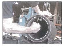
Step 11: Once in place, tighten the ring clamp inside of the CheckMate™ Valve to secure it against the pipe. Using a wrench, tighten the bolts on the clamp until the valve is locked into place. The tightening of the clamp will compress the tape, making it waterproof. When properly done, water will not bypass the seal. If the valve to pipe area leaks, remove the valve and repeat steps 9-10.
