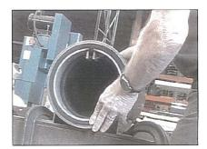
Step 9: Once the CheckMate<sup>TM</sup> Valve has been eased into position, check the O.D. of the valve, making sure it fits snugly into the I.D. of the pipe. If the fit is loose, slide the CheckMate<sup>TM</sup> Valve out of the pipe and apply another layer of rubber tape to obtain the appropriate O.D.
