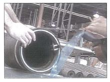
Step 4: Place the rubber tape, adhesive side down, against the outer edge of the clamped end of the CheckMate<sup>TM</sup> Valve. Make sure the edge of the tape is flush with the edge of the valve. Press firmly into place.
