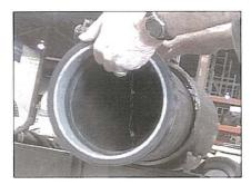
Step 8: The CheckMate<sup>TM</sup> Valve is now ready to be installed into a pipe. Gently slide the valve into the end of the pipe with the clamped end facing out. Make sure the area marked top on the valve is at the 12:00 position. The edge of the CheckMate<sup>TM</sup> Valve should rest flush with the edge of the pipe opening.
