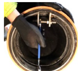
Tightening the clamp compresses the rubber to the pipe
