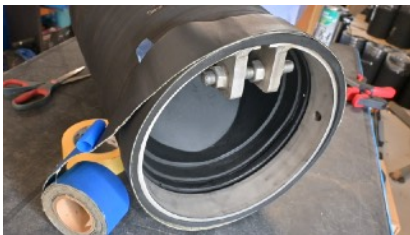
Build out the valve O.D. to match the site pipe I.D.
